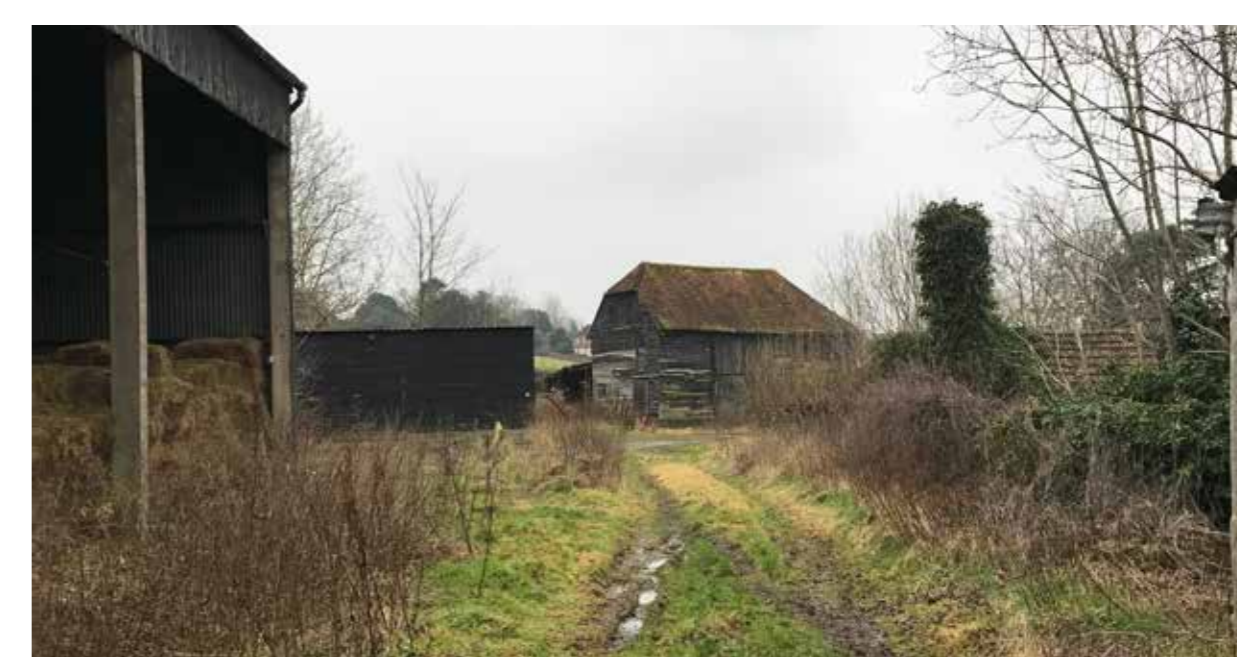
3. View looking south onto listed barn
