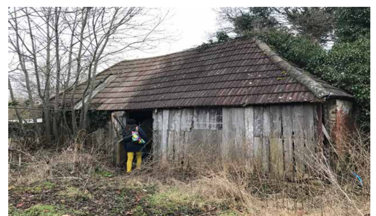
2 Cow shed to be repaired and reused
