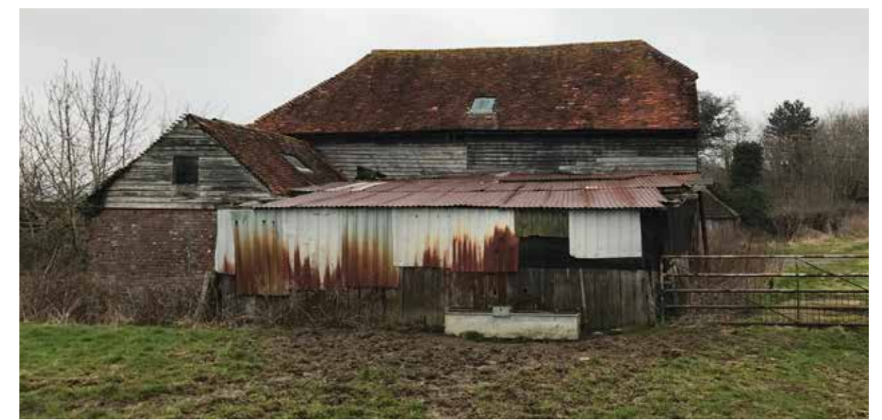
1 Listed barn to be repaired and reused
